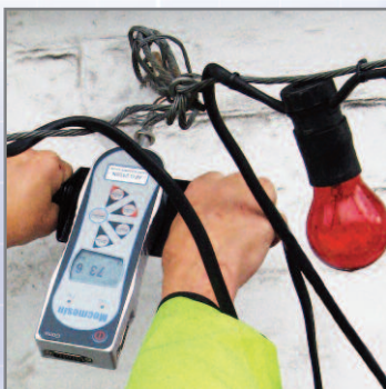
Pull test on anchorage points
